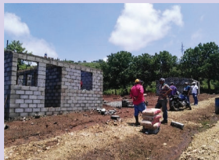
Building a new house in Nueva Jerusalén.
